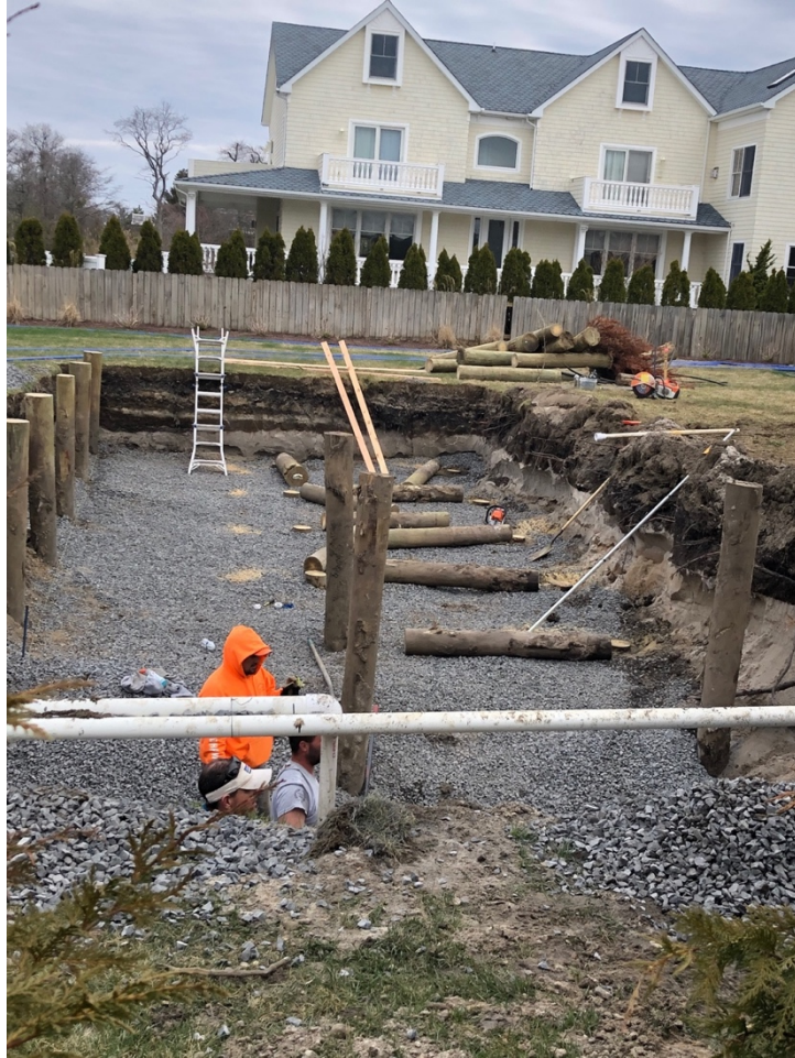
Figure 2: Example of fill on top of sand at 1234 Ocean Ave. (Spring 2019)
