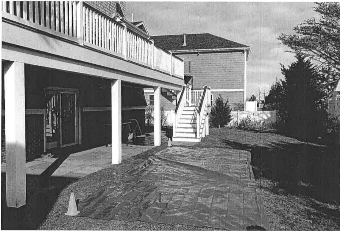
(view facing north)
