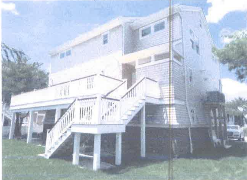
Rear view of 1087 Barnegat Lane 6/24/2015
