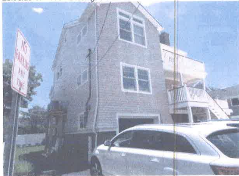
Left side of 1087 Barnegat Lane 6/24/2015
